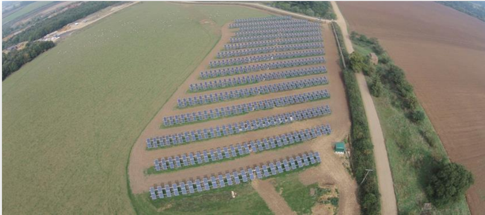
FIGURE 8: LILFORD LODGE FARM SOLAR TRACKER PROJECT
